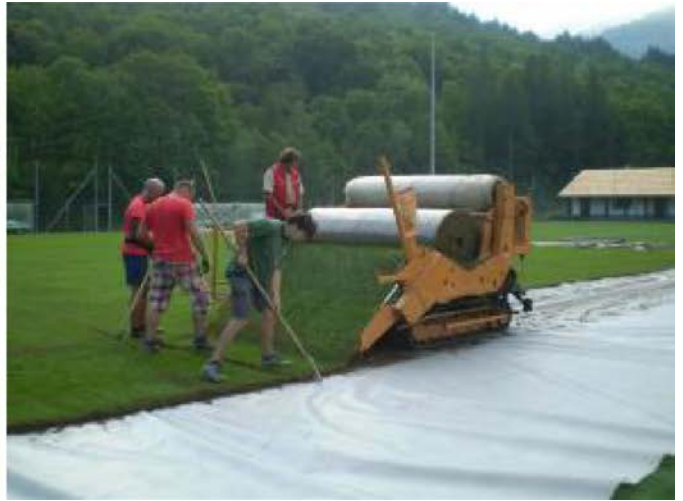
Applying the natural turf upon DuPont™ Typar® geosynthetics; photos by Bruno Marabotto, all rights reserved.
