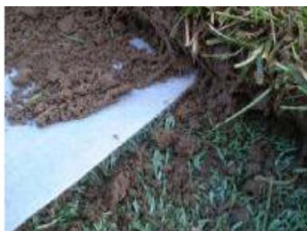
detail of the ground with DuPont™ Typar® geosynthetic applied 施工グラウンド、近接
