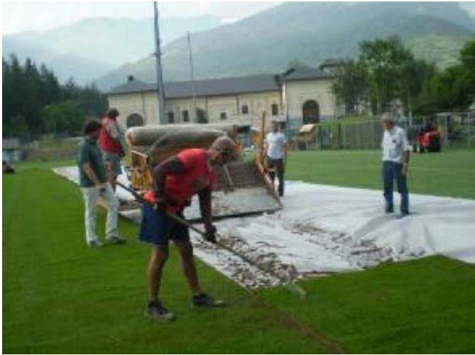
Applying the natural turf upon DuPont™ Typar® geosynthetics; photos by Bruno Marabotto, all rights reserved.
