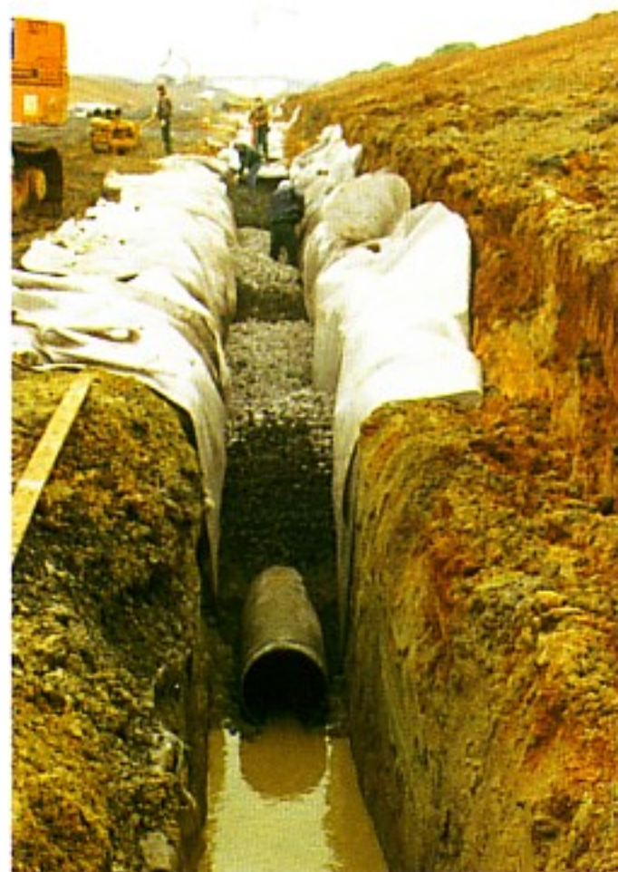
Typar® geotextile used in the trackside drainage helps to filter the ground-water.
