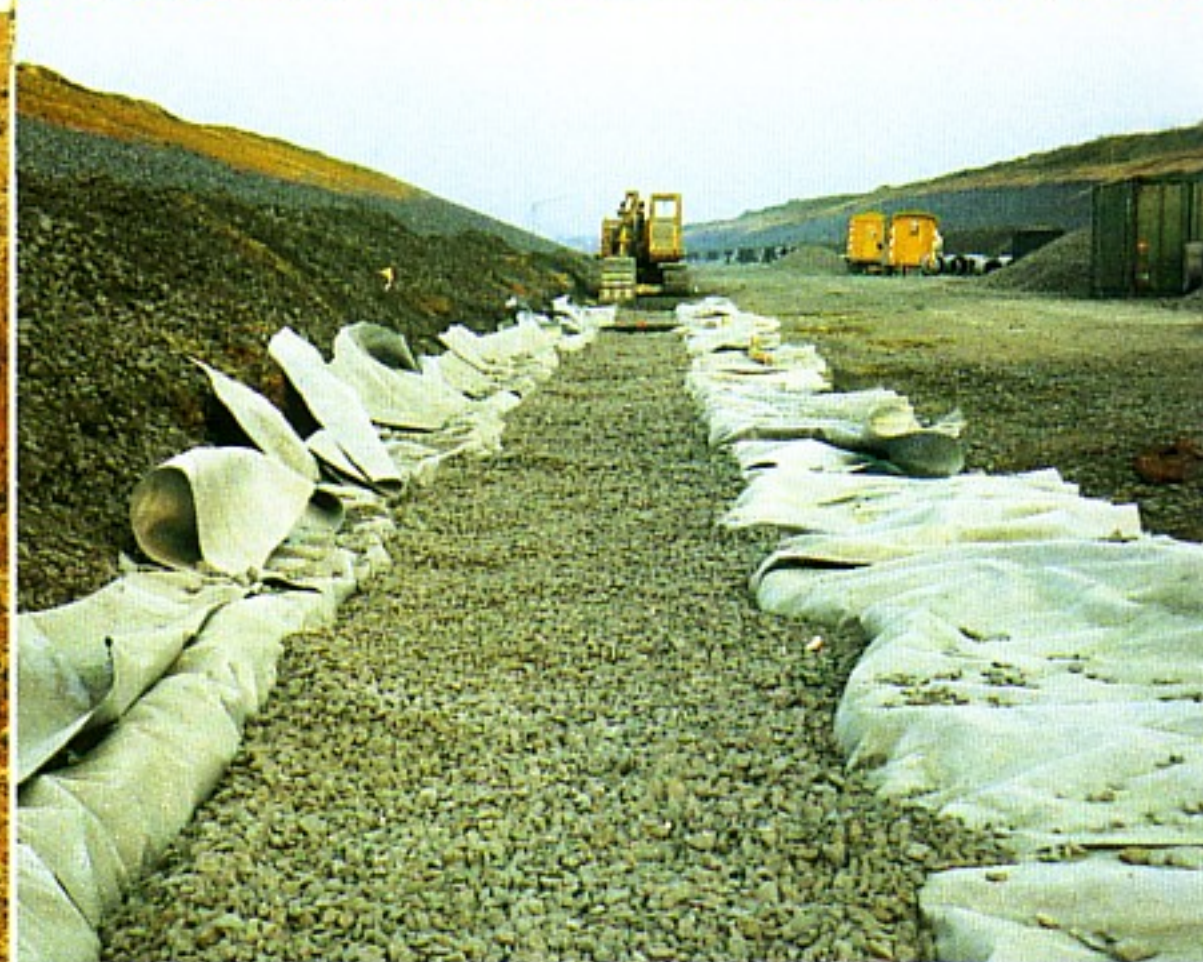
Typar® geotextile used in the trackside drainage helps to filter the ground-water.
